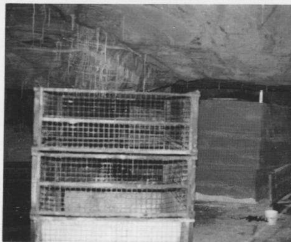
Figure 4. Mesh form and completed support.
